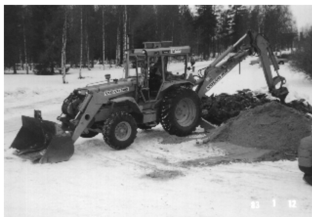
Fig. 1 Tractor excavator (VOLVO BM 616 B)
